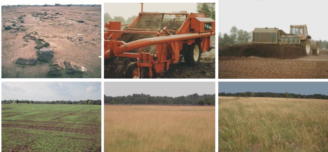
**Figure 19: Example of phytostabilization Lommel-Maatheide (Zn, Cd, Pb) contamination. A: Condition before phytostabilization; B: Removing debris; C: Fertilization; D: 2 weeks after sowing; E: 5 years after sowing; F: 12 years after sowing. Photos Jaco Vangronsveld, UHasselt**
