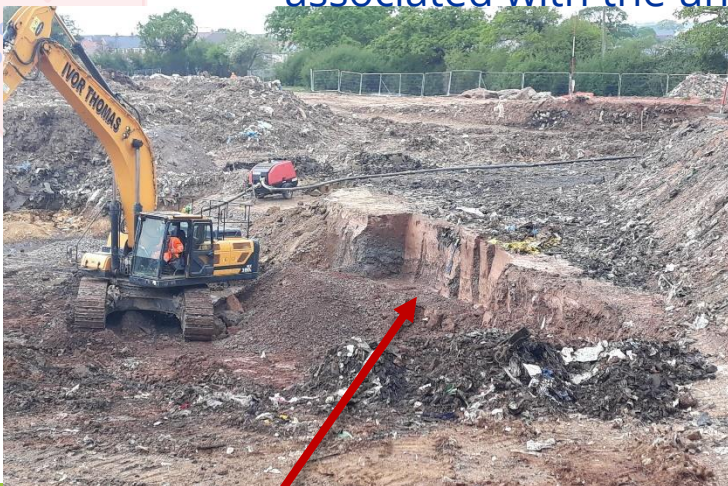
clay stank dividing the waste cells
