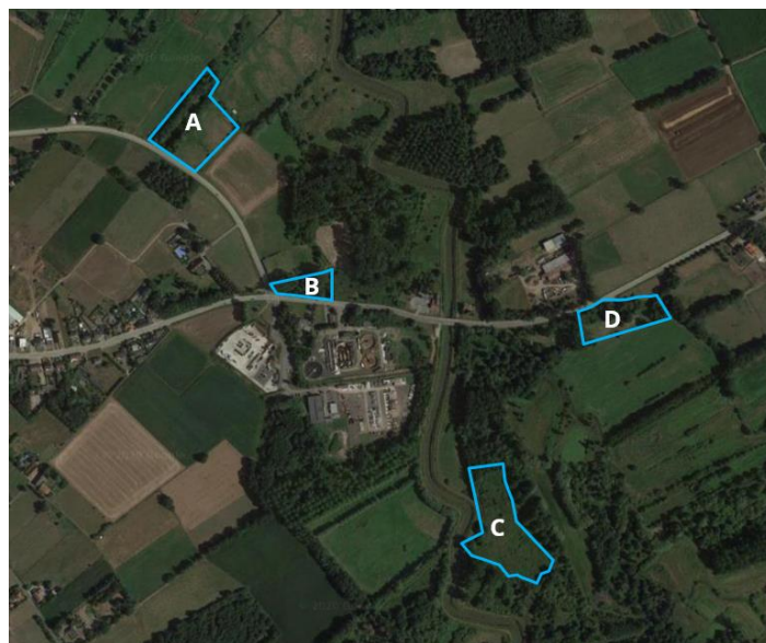
Figure 27: Aerial photograph of the 4 landfills located in the Grote Nete river valley
